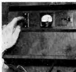
(above) A toggle switch controls elevator car movements. The standby system switch is located to the right of the battery meter.
